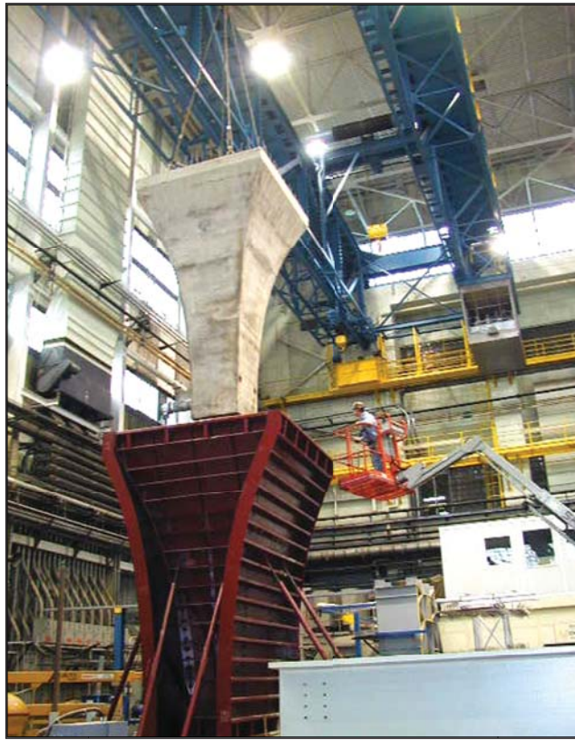
Stripping Concrete Column Form
