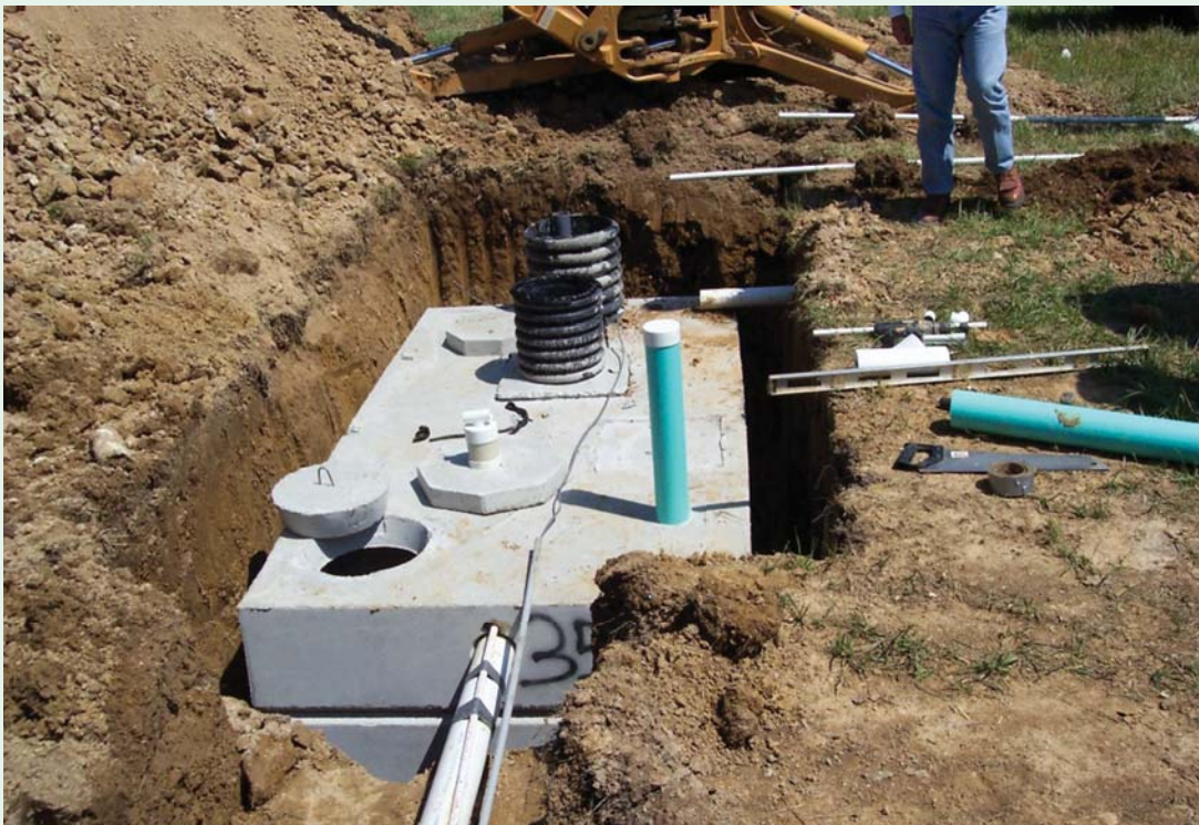
Installation of a H-TWO-O system
