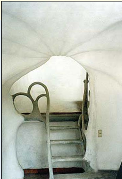
Lower roof and railing, studio.
