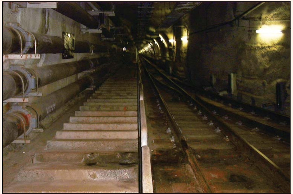
Fig. 5. The inside of Seikan Tunnel.
